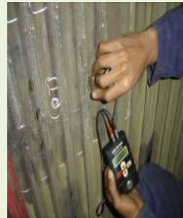
Thickness measurements of water wall tubes furnace
